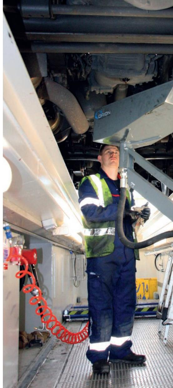
Pits and lanes can both accommodate systems to safely collect used vehicle oils drained out of the vehicle sump, reports Richard Simpson
